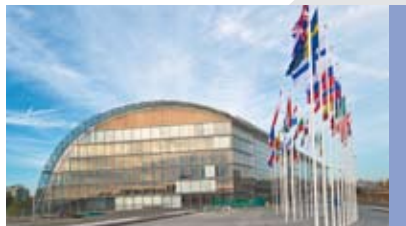
Kirchberg Campus - East Building
