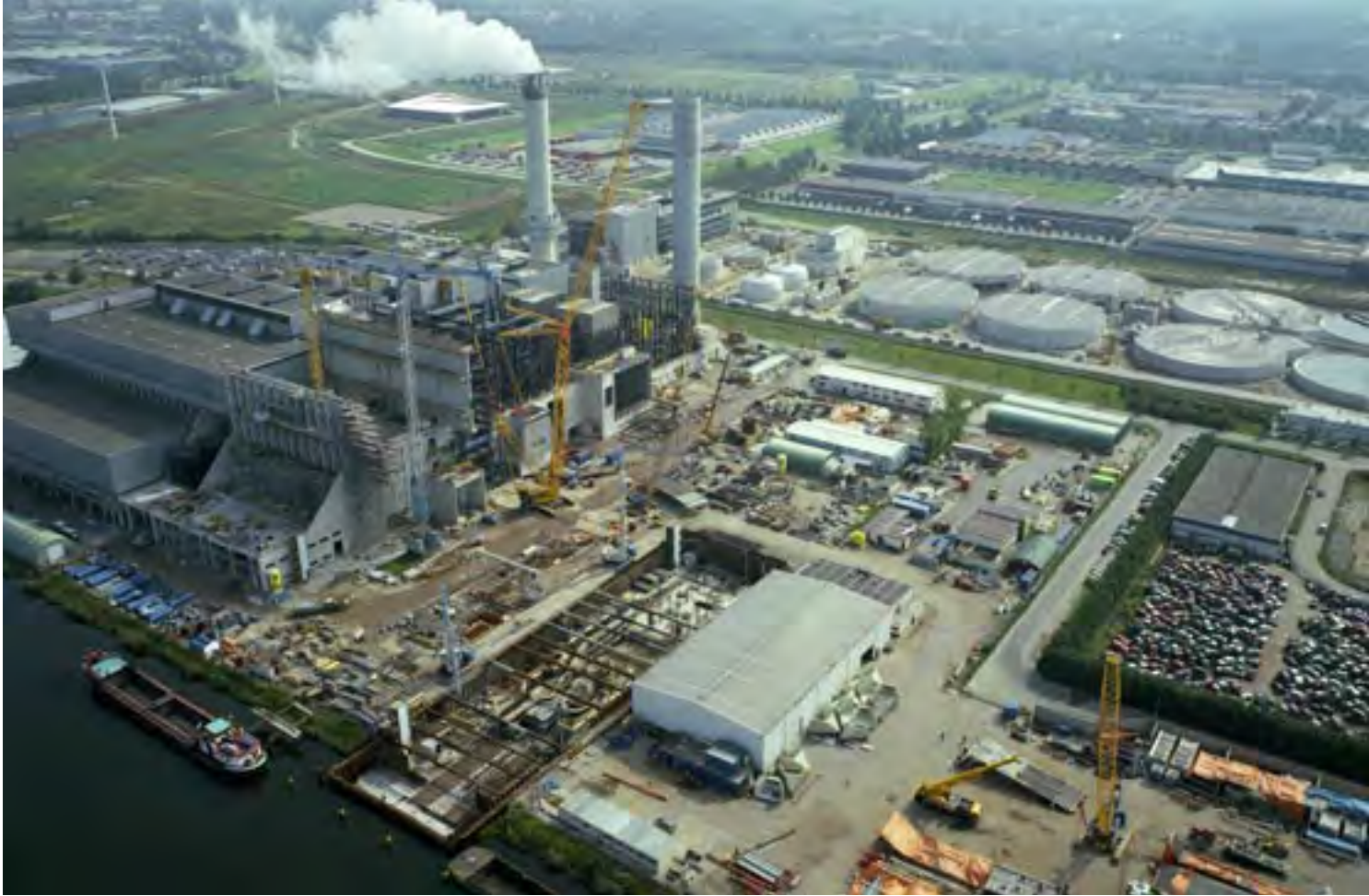
Waste treatment plant in Amsterdam that was built with the help of an EIB loan in 2004. The plant's performance in terms of meeting environmental standards largely exceeds the standards in force in the Netherlands and the EU.
