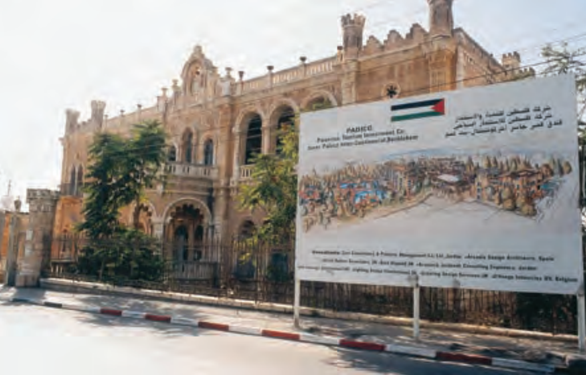
A 250-bedroom international-class hotel co-financed by the EIB in Bethlehem in 1998. Designed to accommodate travellers visiting the Holy Land, the hotel is the first facility in this category in Palestine.
