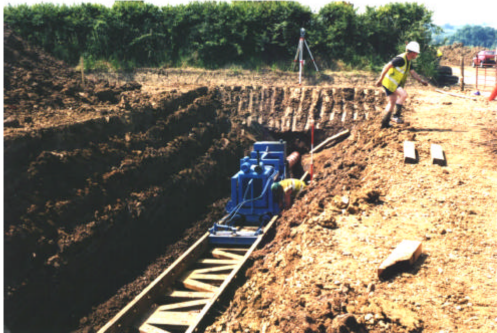
Figure 2.7 – Thrust Bore Machine Being Used at Road Crossing
