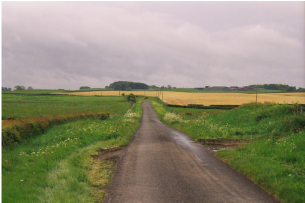
Figure 2.17– Minor road crossing
