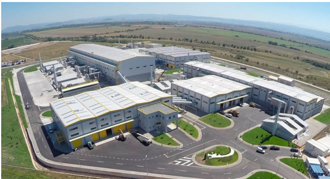
Sofia waste management plant.
