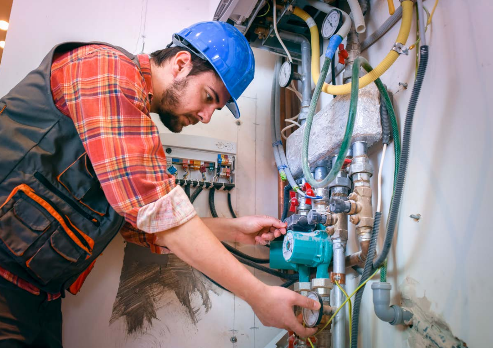
A technician installing a heating system.
