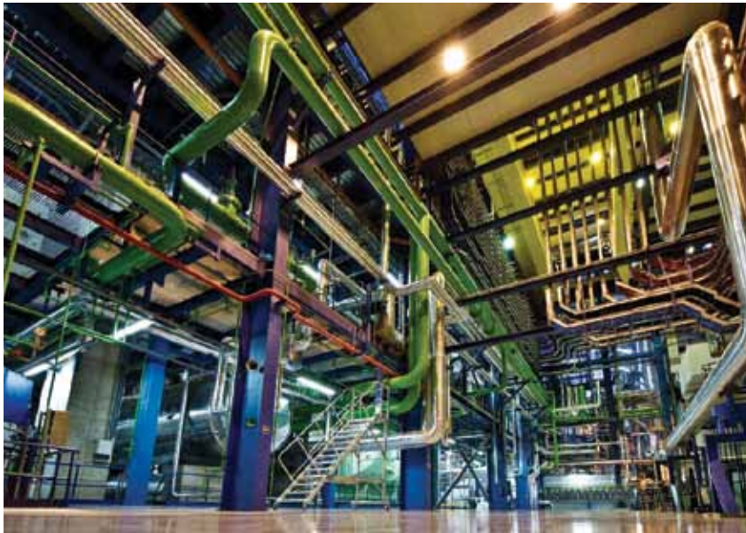
In Latvia, the EIB has supported the upgrading of Latvenergo's combined heat and power plants, as well as its transmission and distribution networks.
