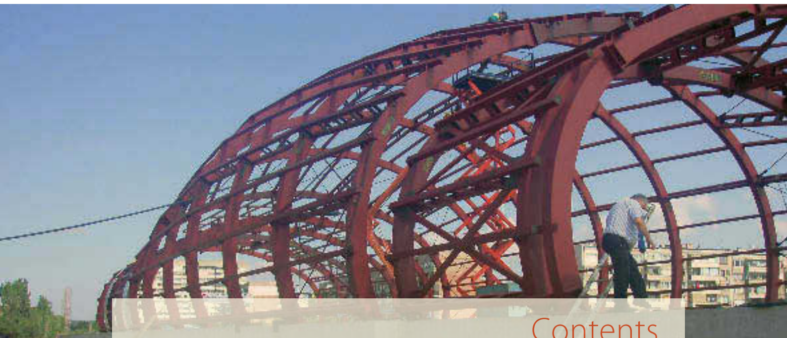
Sofia Metro Extension, Bulgaria
