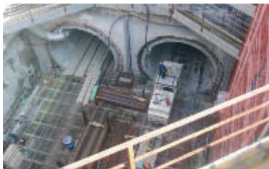
Metro tunnel construction
