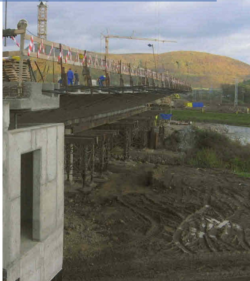
Žarnovica-Šašoske-Podhradie R1 expressway, Slovakia
