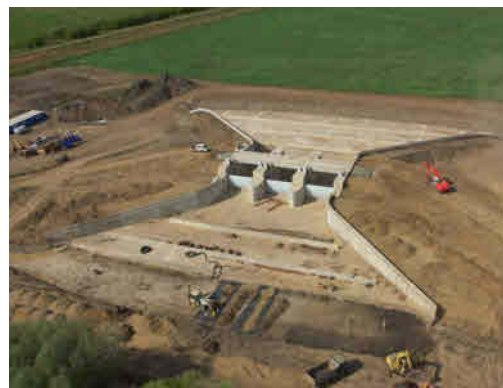
Example of two water reservoir inlet structures
