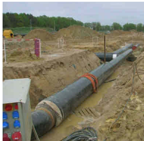
Trench and pipeline construction
