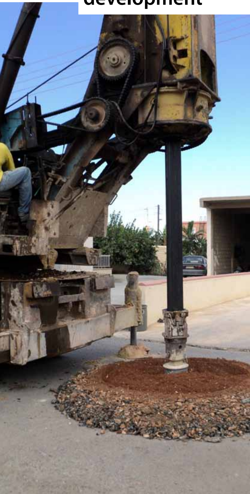
Manhole drilling
