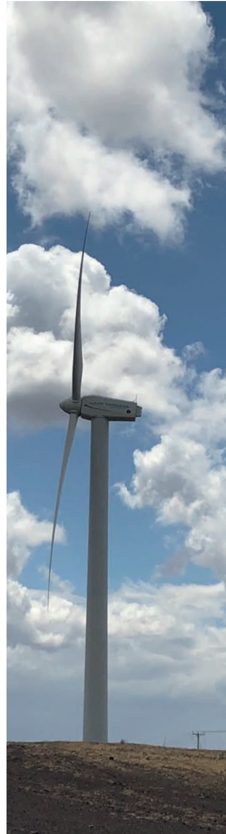
Windpark am Turkana-See
